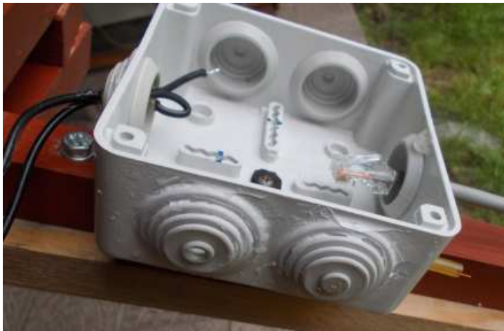
Fig.19 Side caps are sealed with white universal silicone.
