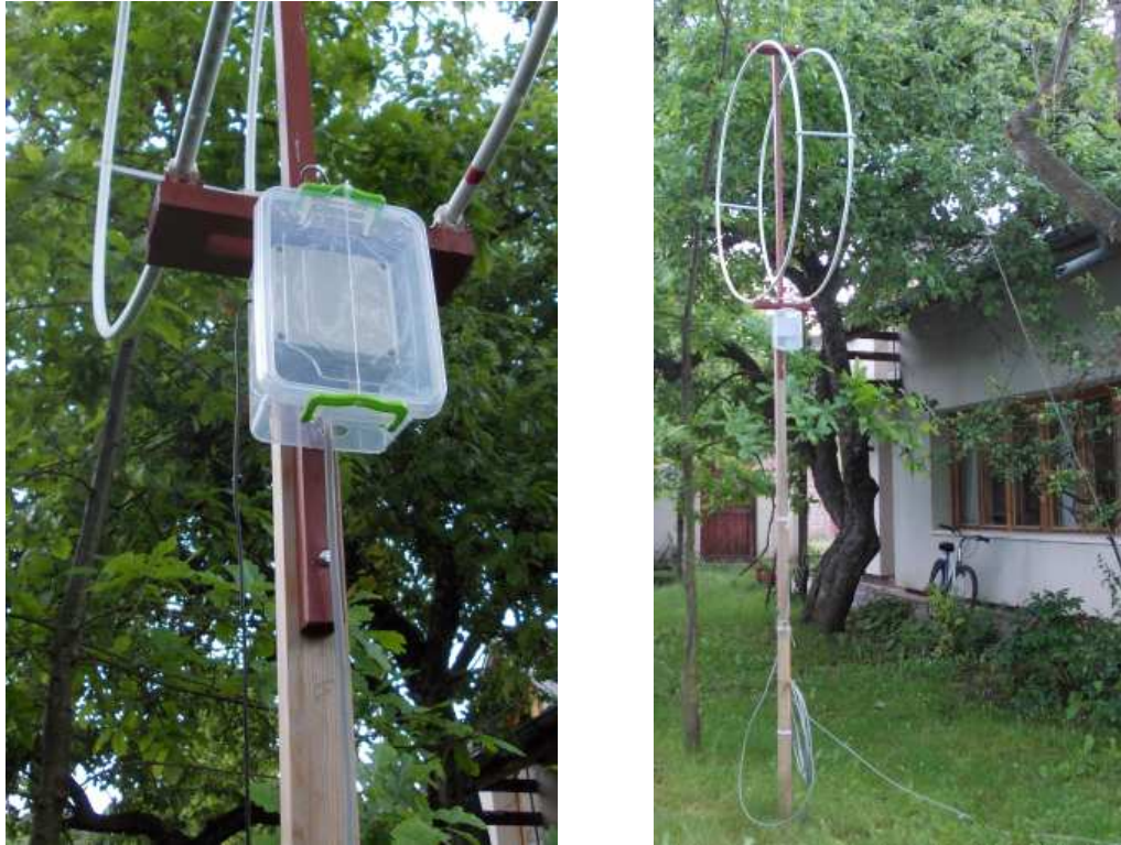
Fig.32, 33 AAA-1 mounted with additional protection box. The amplifier is protected from any rain.
