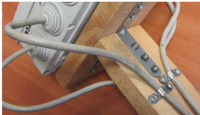
Fig.39 The plank is fixed to the stake by means of two universal clamps. Another clamps are used to fix the FTP cables.
