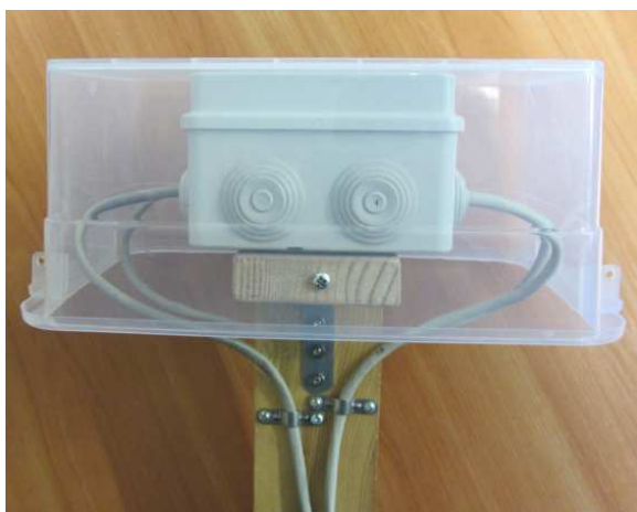
Fig.41 The protection box is fixed upside down with 2 screws to the wooden plank. There is no need to close the box from the lower side. The handles are removed. The possibility for water to enter into the VDLline box is almost zero.
