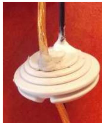
Fig.16 There is no need to seal the lower cap where the FTP cable is passing through. One small hole can be punched into the rubber cap next to the cable hole for a water drainage.
