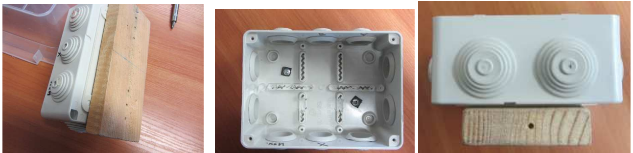
Fig. 35, 36, 37 A wooden plank is prepared which length must be equal to the width of the protective box. A wooden plank is fixed to the VDLLine box with two screws.
