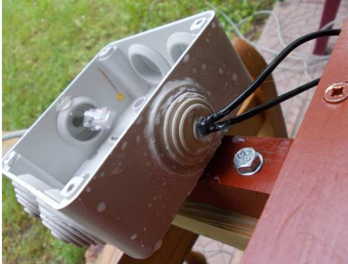
Fig.18 Sealing of the antenna terminals and top cap. This box was inspected immediately after water shower test.
