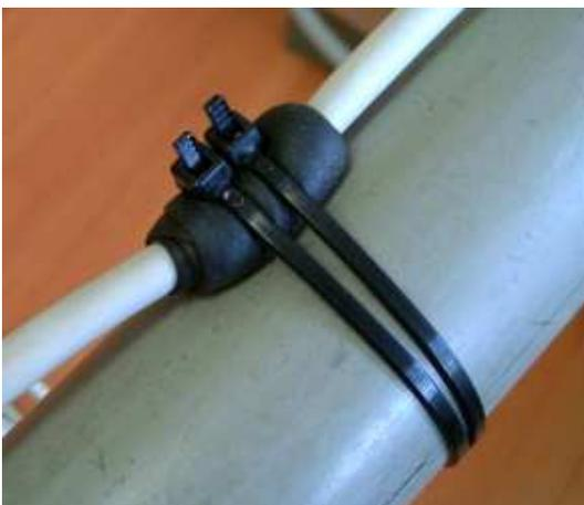
**Fig.4.12** Put several layers of self-amalgamic tape around the cable and fix it with cable ties. Usually the cable shield is made from thin aluminum foil which might be cut if the cable is fasten directly tightly with ties without any protection. Also several layers of cloth tape can be used for this purpose. Even UV resistant ties must be replaced after 1-2 years if they are exposed to direct sun light.
