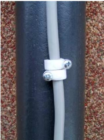
**Fig. 4.11** Using plastic clamps for 6mm cable. These clamps are prepared to be used with nails but 2.9 mm screws can be used instead. Widen the hole of the clamp with 2.9 mm drill. The wall thickness of the PVC tube is usually sufficient to hold the screws tightly. These clamps are very cheap and can be used to fix the cable to its path to the shack.
