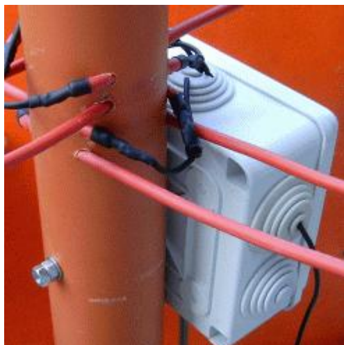
Fig.2.20 Fixing to the mast
