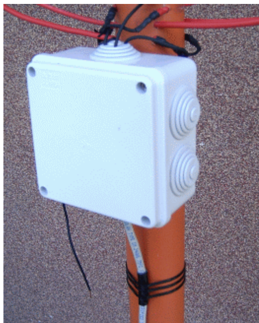
Fig.2.21 FTP cable fixing
